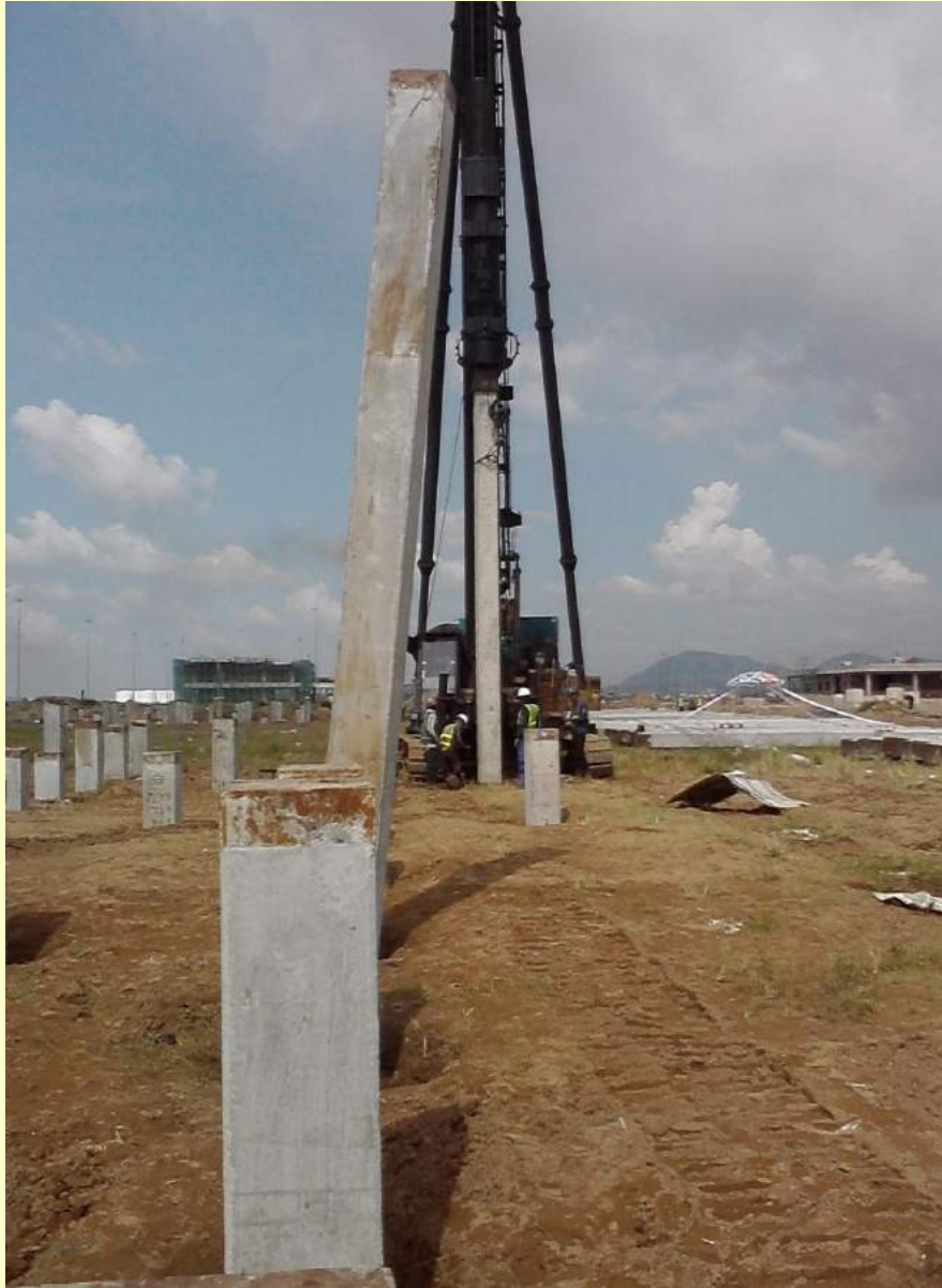
Photos from the driving of piles with extension
